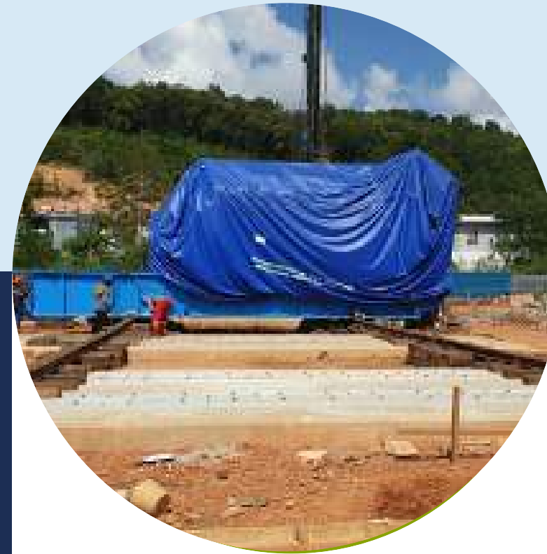
JACKING AND SKIDDING SYSTEM
